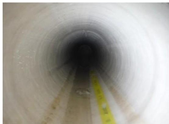
Installed CIPP Liner
